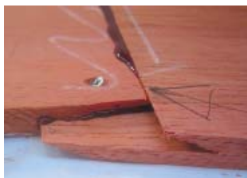
... then driven in at an angle, their smooth shanks help pull the joints together properly.
